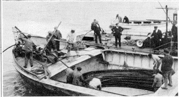
(Top—Right) Passing the Sardinian Shore End from the "Citta di Milano" into a Lighter.
